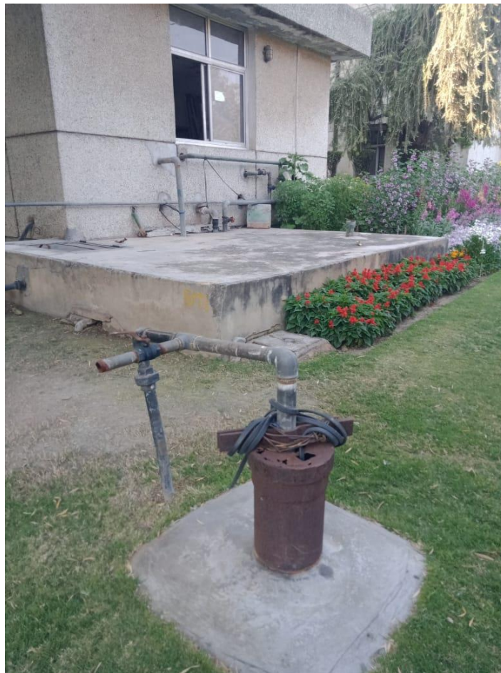
Open well Recharge at International Students' House for Women, University of Delhi
